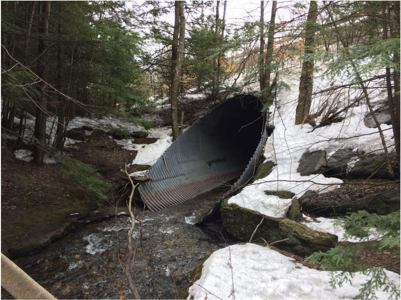
Figure 5. Bridge No. 4 inlet.
