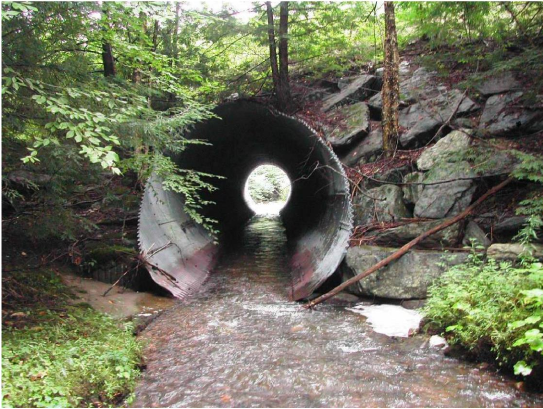
Figure 6: Culvert Inlet
