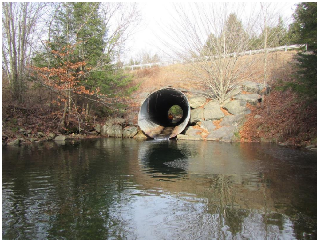
Figure 6. Bridge No. 4 outlet.
